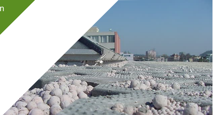
FLAT ROOF INSULATION
